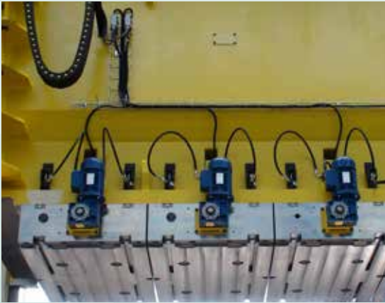
Pull cylinders on a large slide with parking stations
